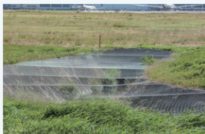
▲ 機場內水溝設置防鳥網。 Bird-control nets installed over drains inside the airport.
