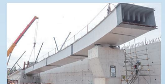
▲ 航站北路鋼樑吊裝施工。 Erection of steel beams on Hangzhan North Rd.
