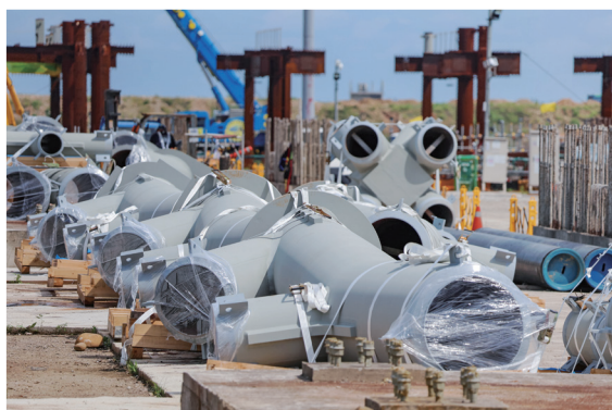
▲ 待吊裝的巨柱鋼構組件。 Structural steel components ready for lifting.
