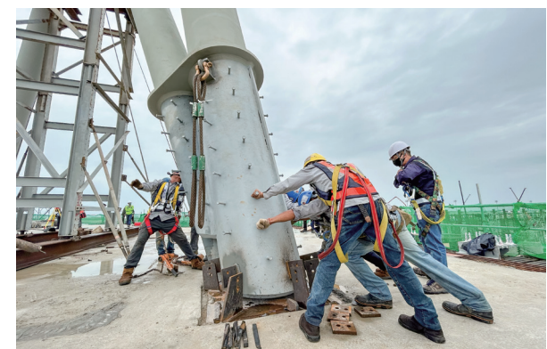
▲ 技師們在第三航廈工區進行吊裝作業。 Engineers conducting the column-lifting operations at Terminal 3 construction site.
